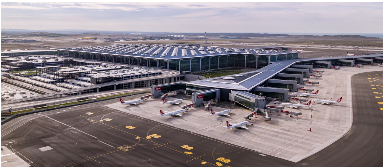
Fig.10: Istanbul Airport: World’s First Solar-Powered Airport [62]
